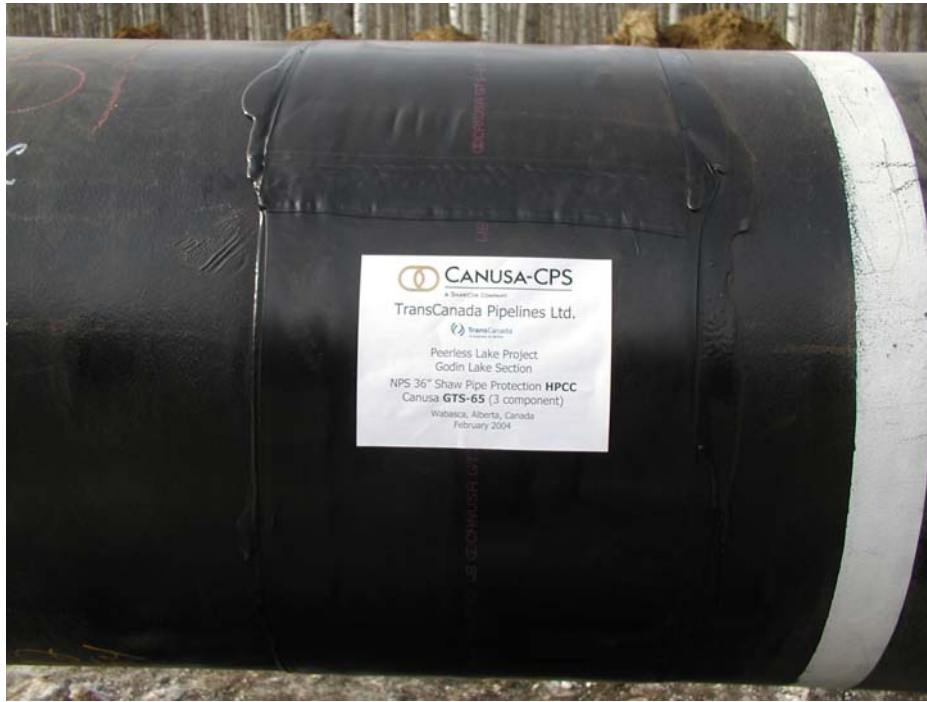
Figure 3 Canusa GTS-65 three layer heat shrink sleeve on a field joint.
