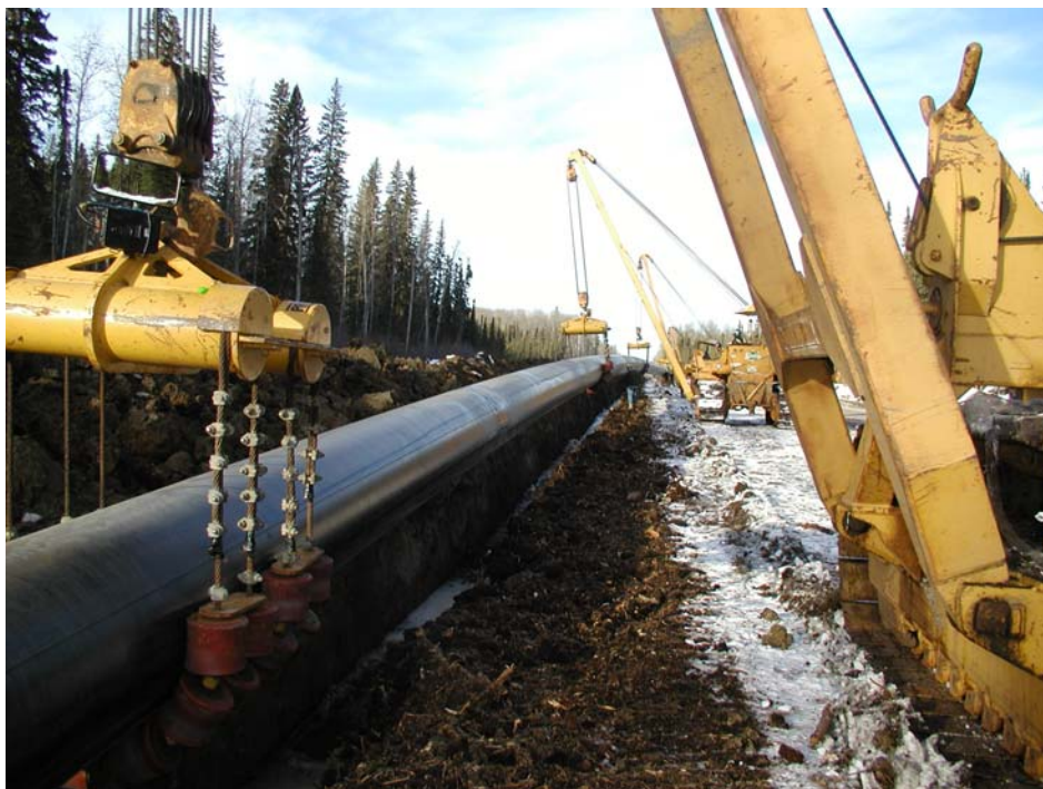
Figure 4 Lowering in of pipeline.
