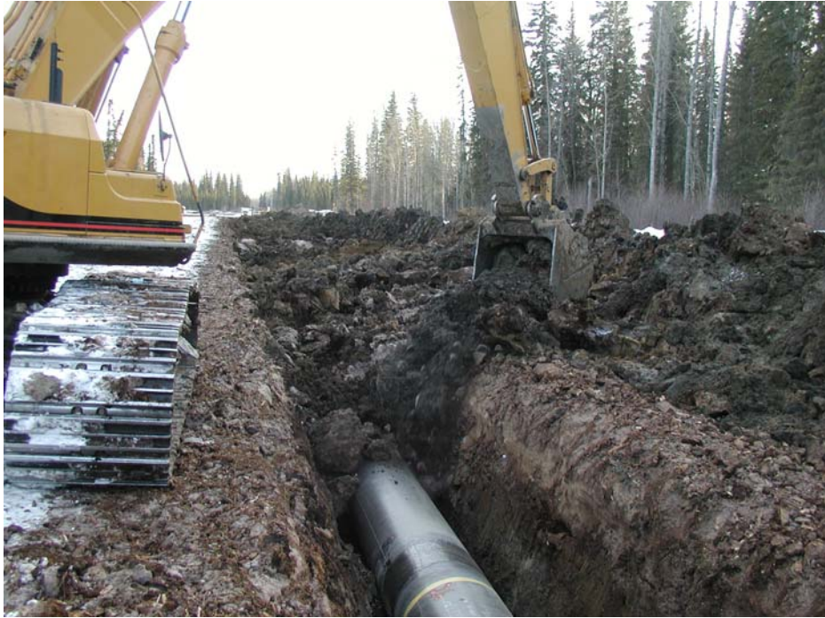
Figure 5 Backfilling of pipeline.
