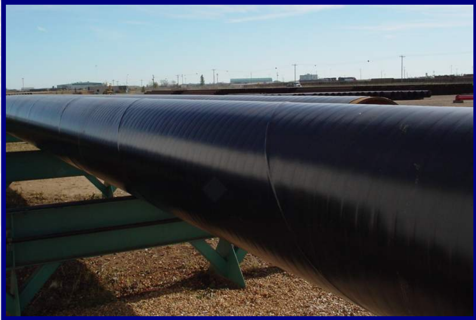
Side-Wrapped GSPE on Spiral Weld Pipe (30")
